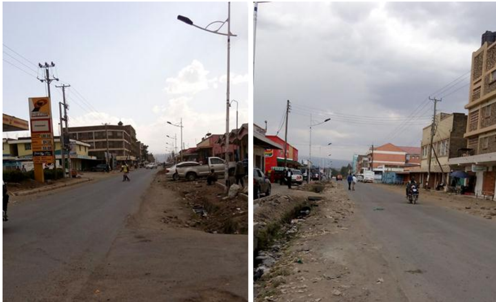
Figure 53: Existing Conditions along Kanu Street
